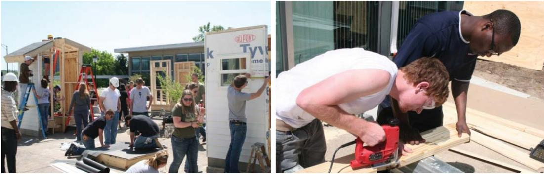
Figure 4: Project 2 Build Day – Left the Groups in Various States of Construction; Right N. Bosman and D. Ojo Cut a Birdsmouth Notch.
